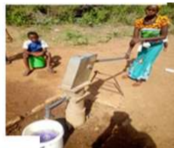
Plate 1 D: Kanmonu hand pump borehole
